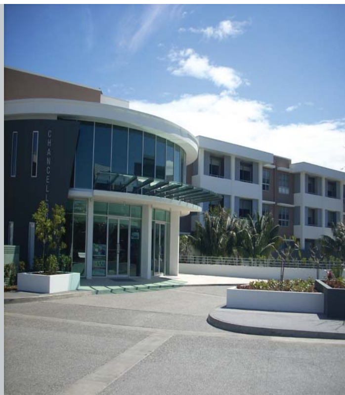
'The Chancellor', Varsity Lakes Gold Coast, comprising 64 units and 3700m 2 of commercial space. Units sold out prior to completion.
