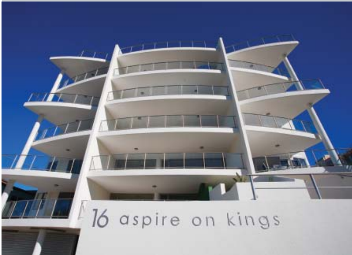
'aspire on kings', 15 units overlooking Kings Beach, Caloundra. Constructed on time and within budget with a steady sales rate. Loan now repaid.
